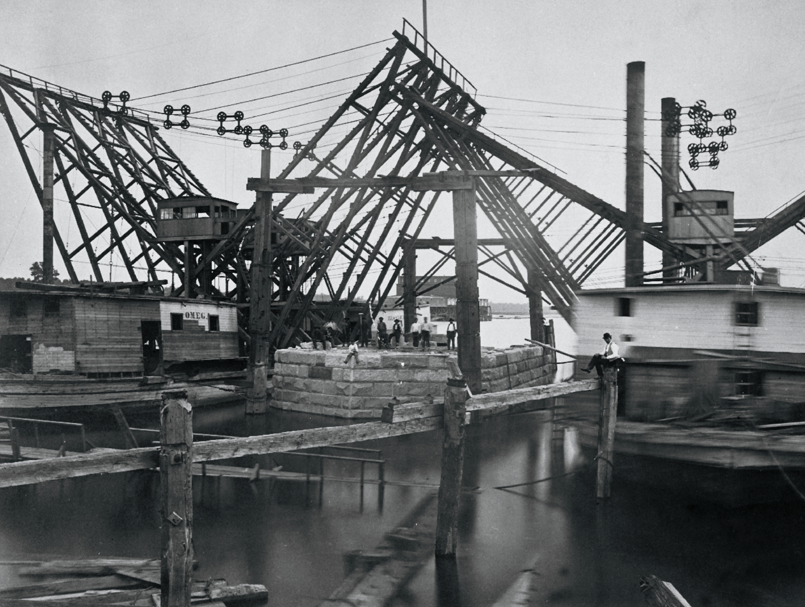
This view shows the two pontoon boats, Alpha and Omega , building the west pier. Stone laying is well advanced, forcing the iron caisson down into the riverbed. Robert Benecke; Missouri Historical Society
