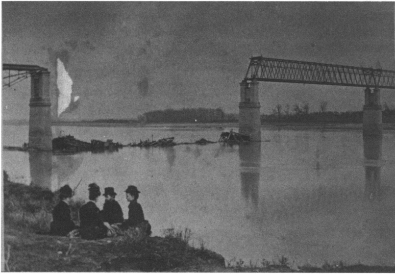
FIG. 7 A lovely spot to picnic and to contemplate mortality. Image of the St. Charles Bridge after a derailment brought down one of its 318-foot-long Warren trusses. It is unclear whether this is the 1879 event when five men died and eighteen cars dropped into the river, or the 1881 collapse that resulted in the loss of thirty-one cattle and freight cars and the death of the locomotive engineer. In each case, the company simply rebuilt and carried on. (Source: "Wabash—First Missouri River Bridge" [photo 2], Bridgehunter.com, available at http://bridgehunter.com/mo/st-charles/first-wabash-rr/ [accessed 2 May 2012].)
