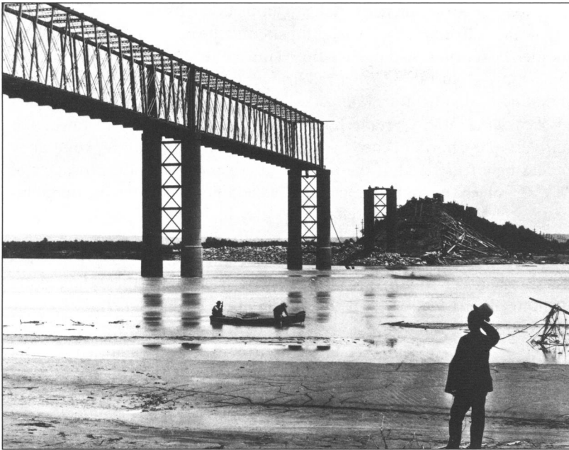
FIG. 8 The Union Pacific Railroad crossing of the Missouri River at Omaha had Post trusses on iron pneumatic piers. The bridge lost two spans to an 1877 tornado. Ferries provided a temporary and unsatisfactory substitute while the railroad replaced its errant spans—in just six weeks. In 1886–87, the Union Pacific built a new double-track Omaha bridge on new masonry piers. By 1916, it put up even stronger spans here to support heavier loadings. (Source: “Union Pacific’s First Bridge,” image BF14-236, Bostwick-Frohardt Historic Omaha Photo Collection, folio 14, negative 236, Durham Museum, Omaha, Nebraska, available at http://durhammuseum.contentdm.oclc.org/cdm/singleitem/collection/p15426coll1/id/1686/rec/1 [accessed 3 May 2012].)
