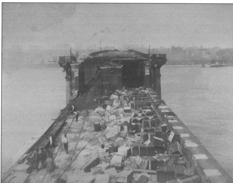
FIG. 10 This westward-facing photograph (St. Louis is on the far shore) shows the remnants of the stone arcade that once supported the roadway deck shown at left in figure 1. As depicted here, the 1896 tornado blew off a section of the roadway, tumbling its supporting stonework across the bridge's railway deck. Eads's steel arches remained largely unscathed. (Source: Author's collection.)
