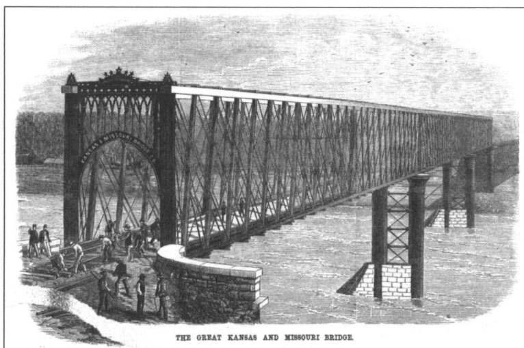
FIG. 6 The Leavenworth Bridge in 1873. Note the Post trusses and pneumatic tube foundations, reinforced with cut stone to protect against strong currents and ice floes. Common roadway traffic used this bridge when trains were not scheduled to cross. For St. Louis, Boomer and Post planned this basic configuration for the piers, but with two additional trusses in each span, allowing a full separation of roadway and rail traffic. (Source: Image, "Bridge over the Missouri River," Scientific American , 15 March 1873, 167, reprinted by Bridgehunter.com, available at http://www.bridgehunter.com/ks/leavenworth/fort-leavenworth/ [accessed 1 May 2012].)
